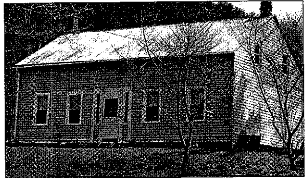
John (1816-1866) and Lydia Teator's house Rt 145, Schoharie Co, Livingstonville
